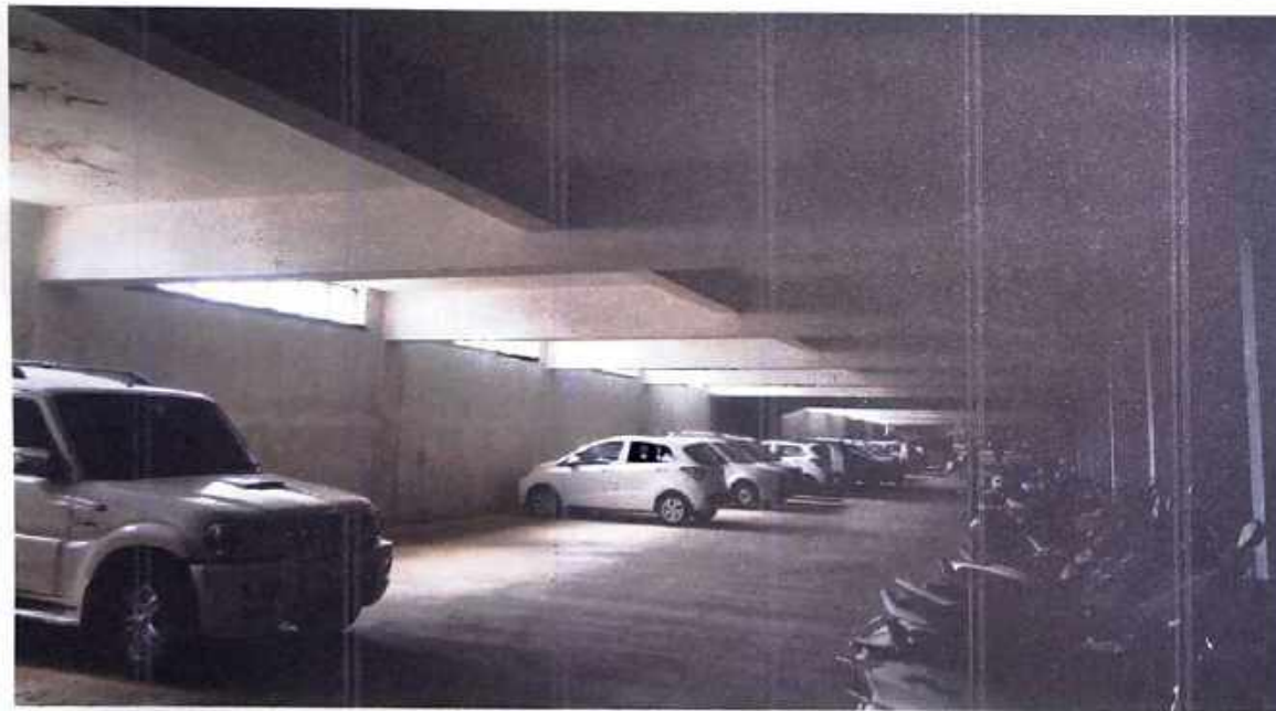
Basement Parking with daylight penetration and natural ventilators to exhaust smoke.
